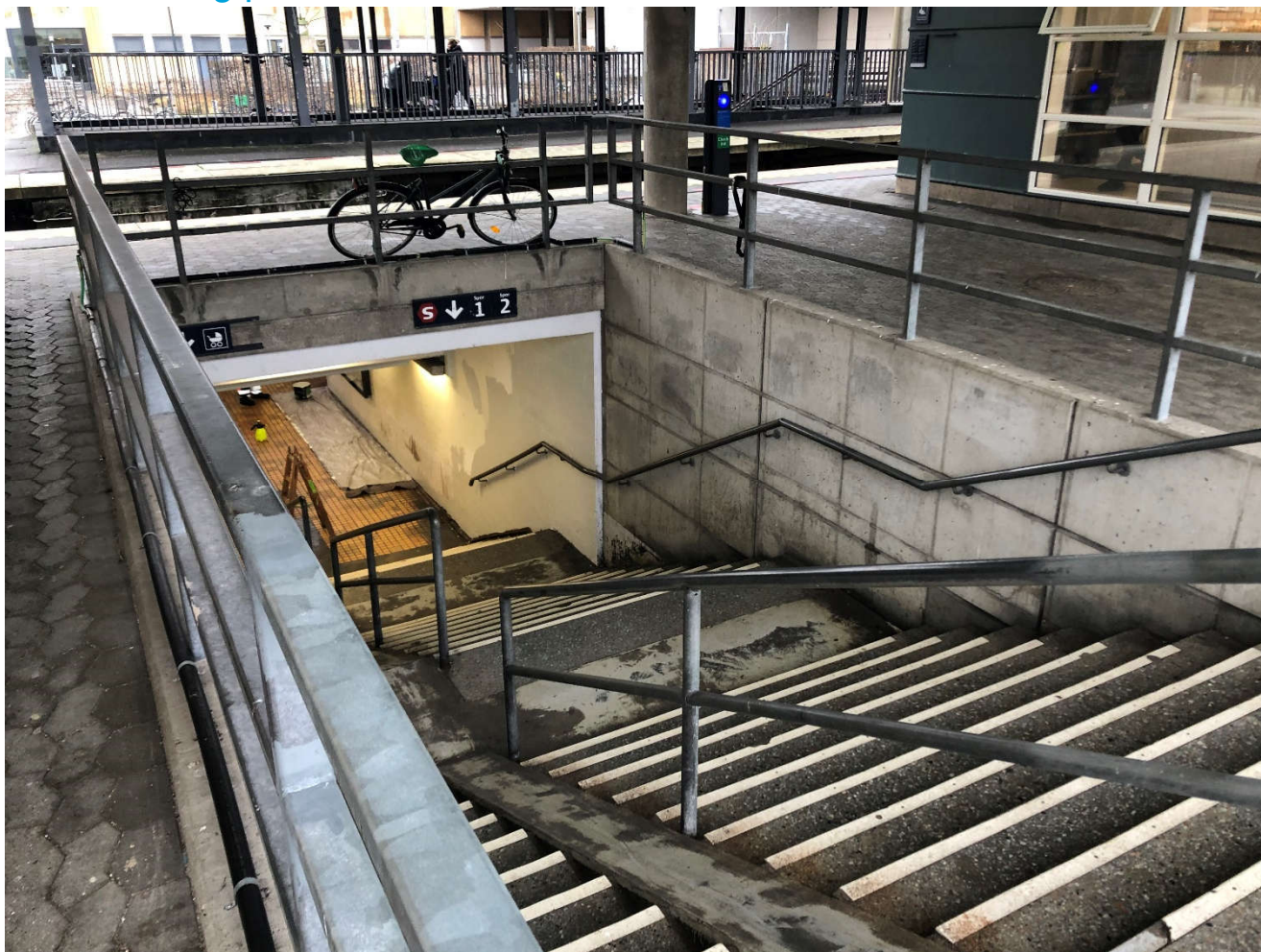
Figur A-1 - Ballerup station – Trappen nord for banen
